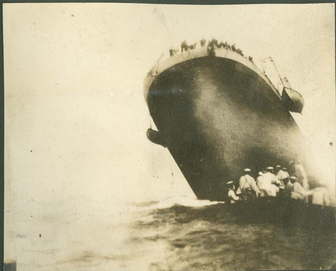
Bow of S.S. City being taken down 3 rd day by crane from Tacoma Cruise Kasuga
