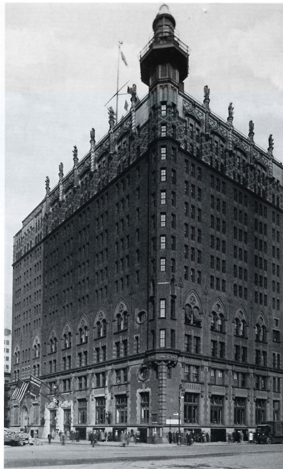
The SCI building at 25 South Street with Titanic Memorial Lighthouse at the top.
