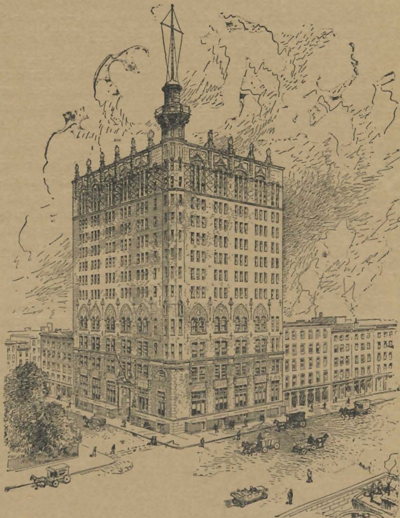
NEW BUILDING Now being erected
