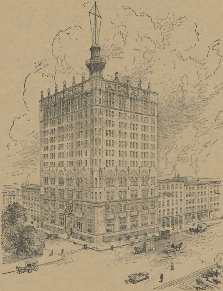
NEW BUILDING Now being erected
