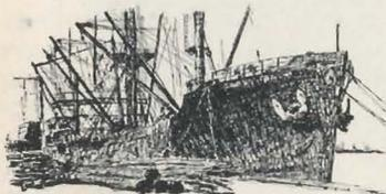
Freighter: the hull is divided into a number of large compartments called holds in which cargo is stored. Cargo is hoisted into ship by its winch and boom arrangement which can lift up to 50 tons.
