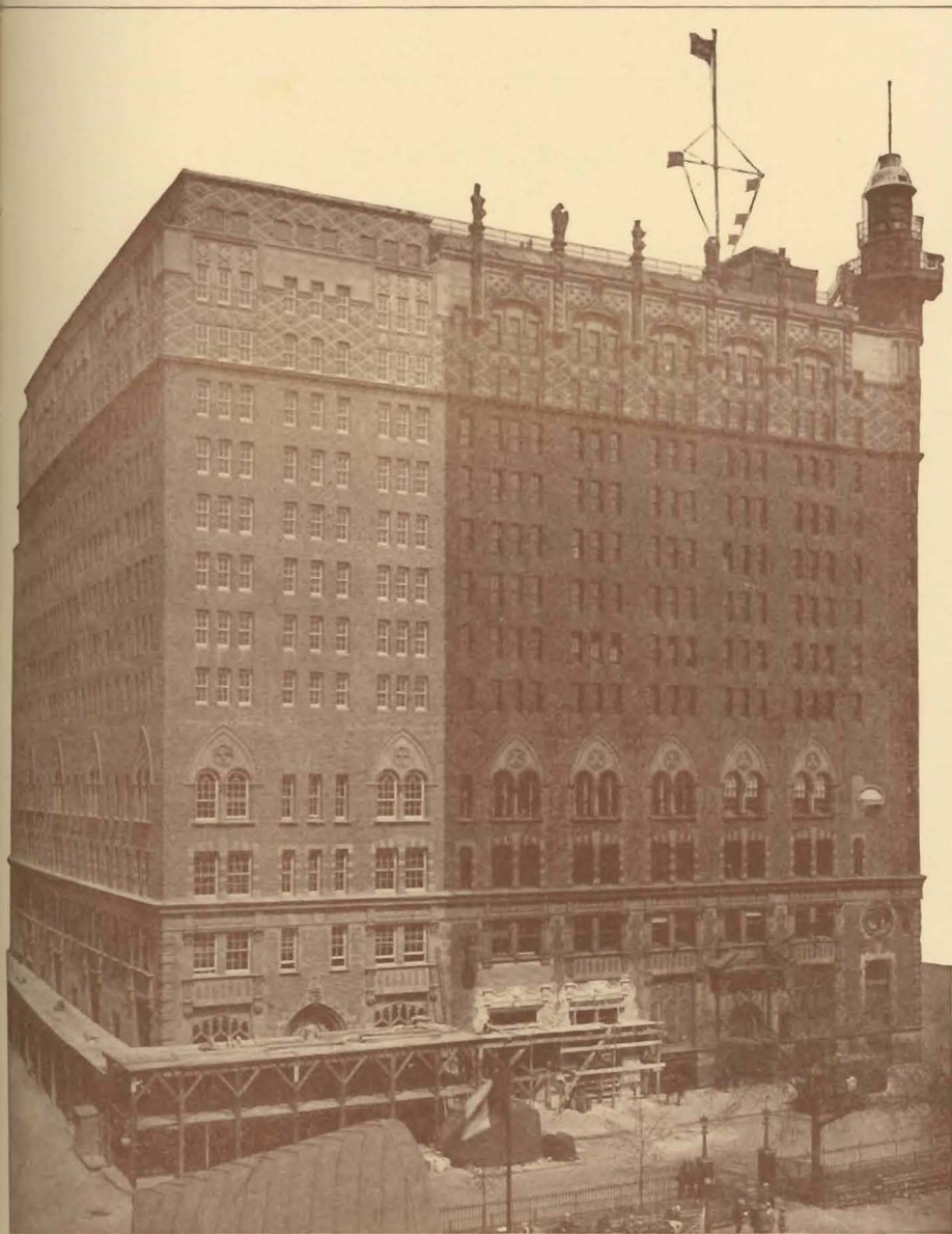
Present status of new Annex construction
