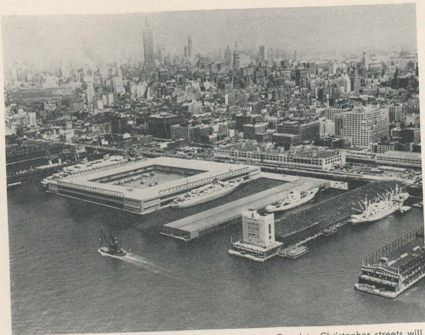
New York waterfront, 1958: The North River docks, from Canal to Christopher streets will look like this in 1958, when Holland-America Line moves to New York City.
